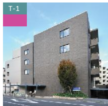
KDX Daikanyama Residence
